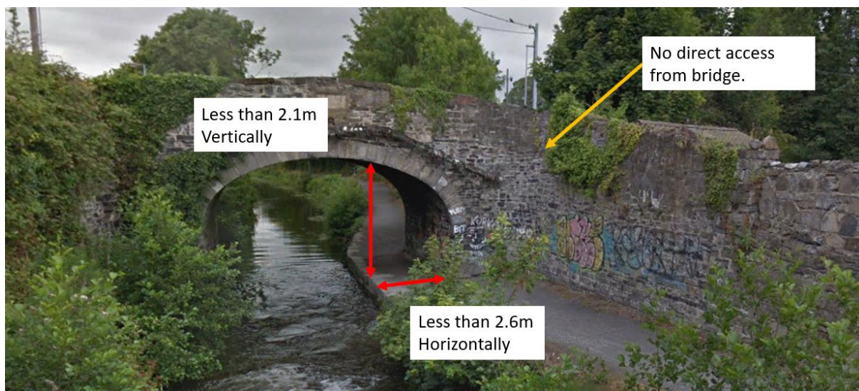
Figure 2-5 East elevation of Clonsilla Road Bridge showing limited access.
