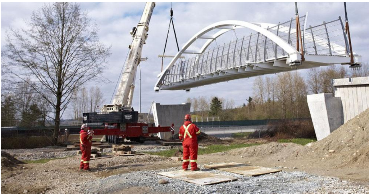
Figure 3-5 Typical Bridge Lifting Operations (One Lift)
