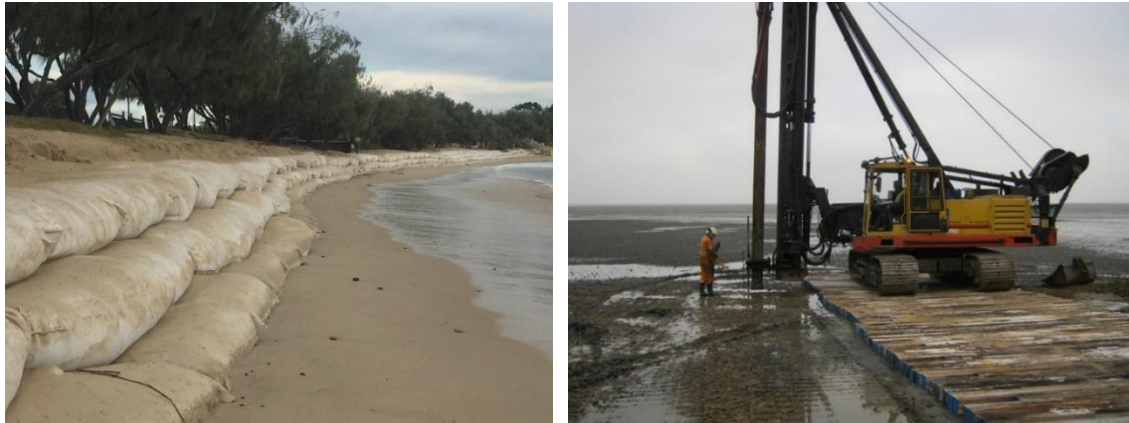
Figure 3-3 Typical Geotextile Filled Bags and Timber Piling Mat (Temporary)
